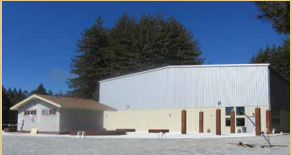
A view of the new gym and bathroom building nearing completion
